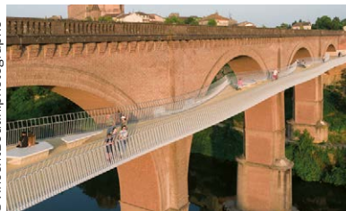
Footbridge Albi France
